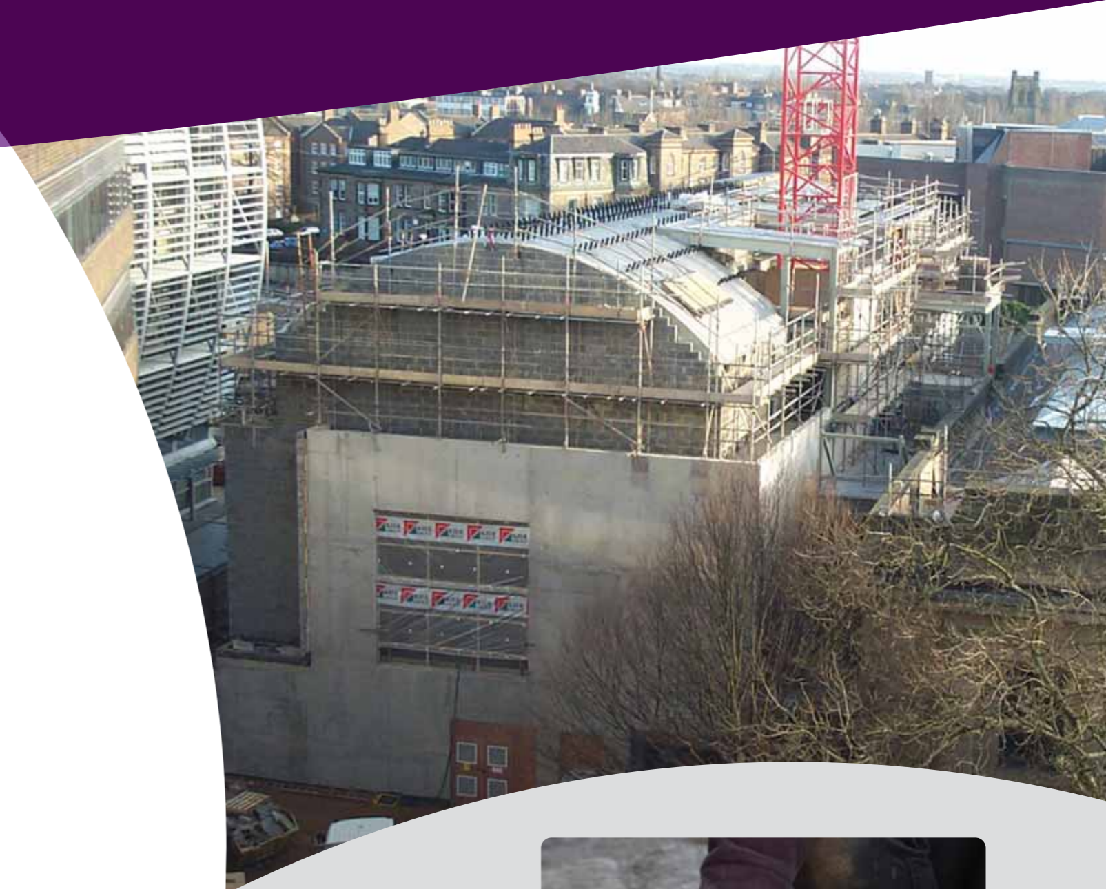
Above: rear extension of the Great North Museum project.
