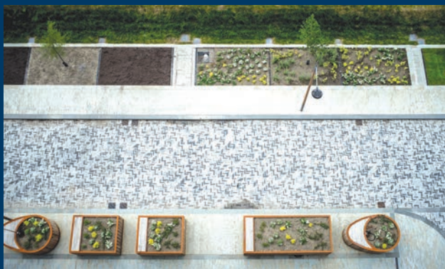
Sustainable Drainage Systems Facility and Demonstrator (SuDS) at the Urban Sciences Building
