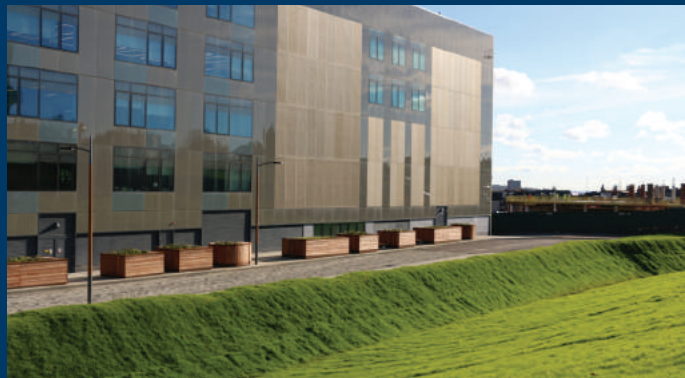
Sustainable Drainage Systems Facility and Demonstrator (SuDS) at the Urban Sciences Building
