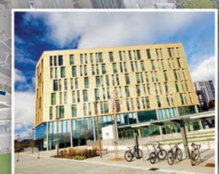
4) The Core Completed: November 2014
