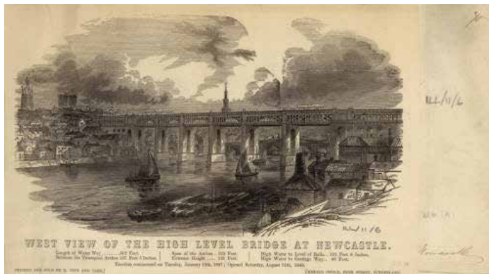
West View of the High Level Bridge at Newcastle
