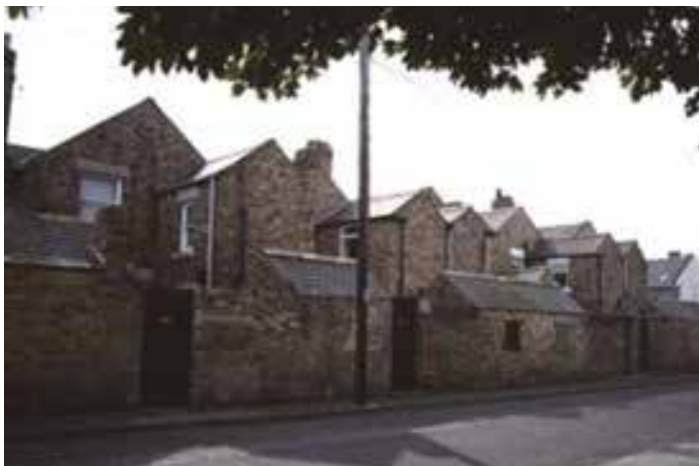
Reference: Photograph of Nos 15 To 19, With Backyard Walls And Outbuildings © Crown copyright. Historic England Archive. IOE01/14603/29
