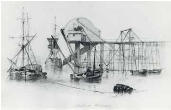
Etched print of a landscape view of collier boats being loaded at the Wallsend drops
