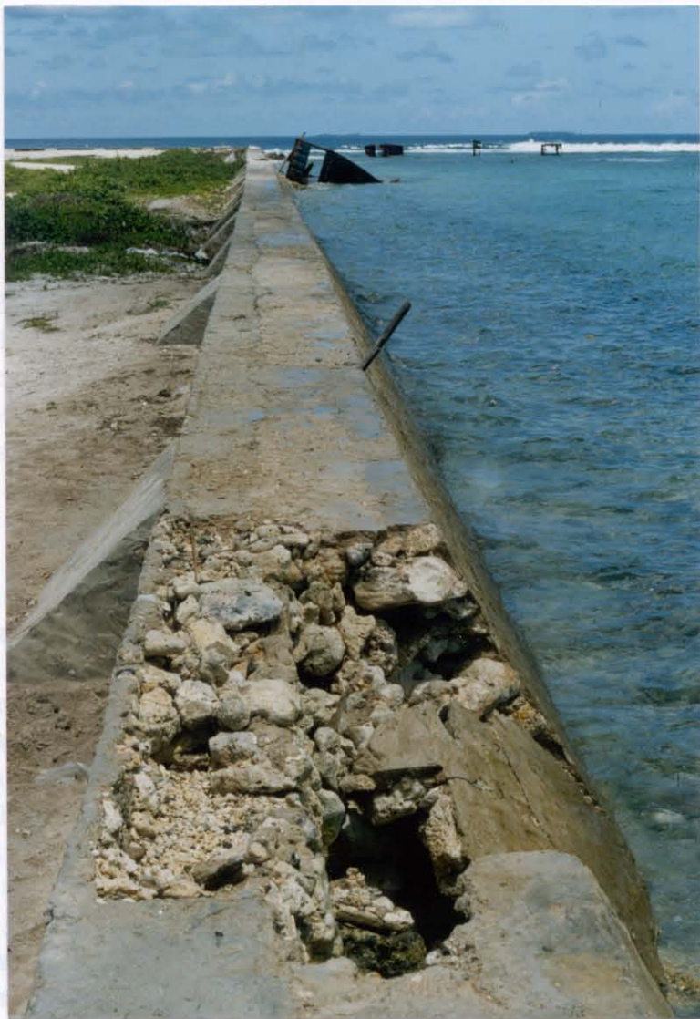
FIGURE 39. Part of the retaining wall on the south-west of Hulule (marked C on Fig. 19). This traditional design wall appears to have been undermined leading to collapse from within.
