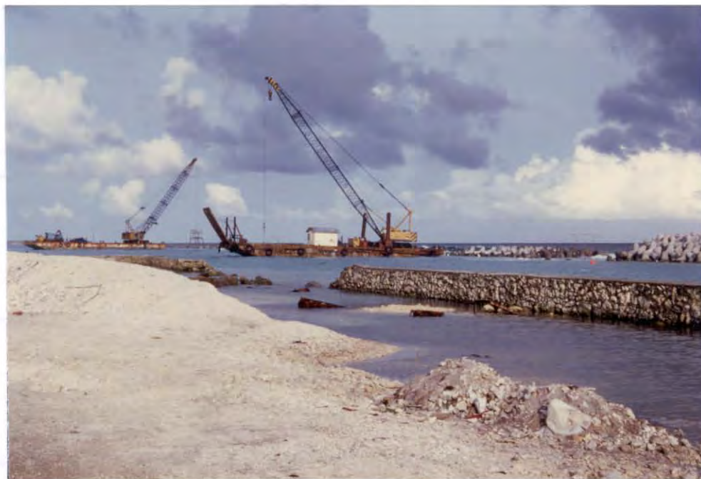
FIGURE 34. Edge of the reclaim area on southern Male' Island, showing damaged retaining wall, lost infill and work in progress on the construction of the detached breakwaters to protect the reclaim.
