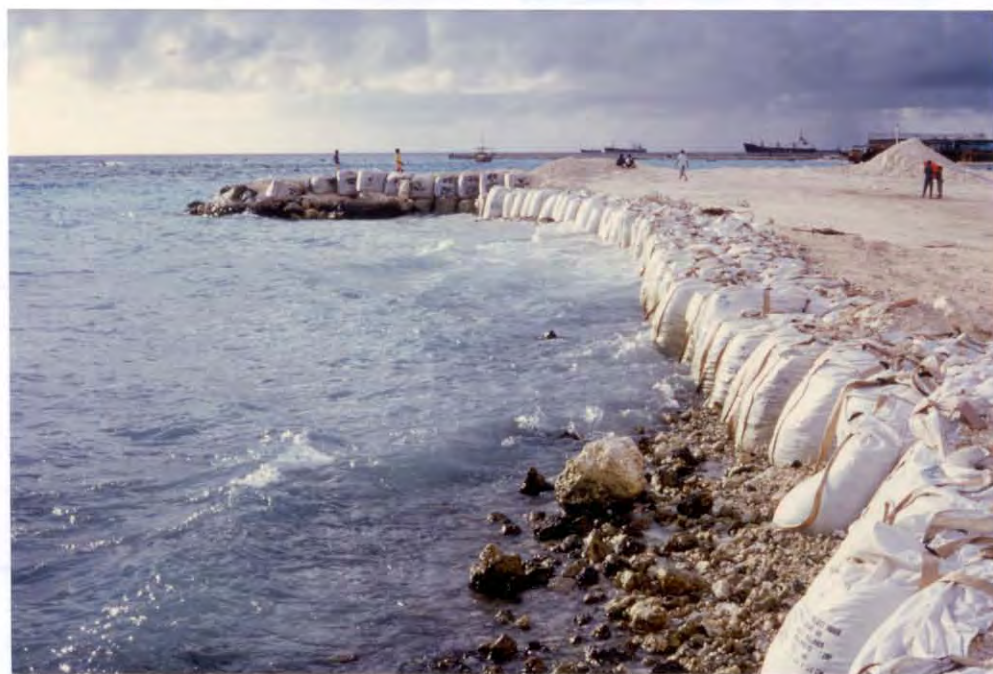
FIGURE 35. South-west coast of Male'. This area will eventually be protected by the breakwater enclosing the proposed port here. Currently, shore protection is provided by these sacks of coral rubble.
