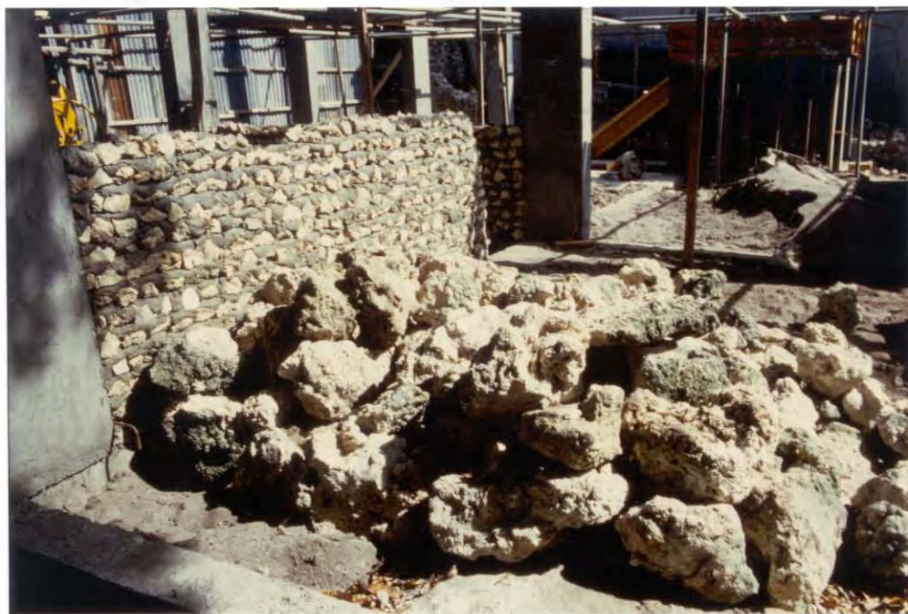
FIGURE 28. A pile of coral blocks mined from the reef flat at a building site in Male'. An internal coral wall is in the process of being built from broken up pieces of these blocks.
