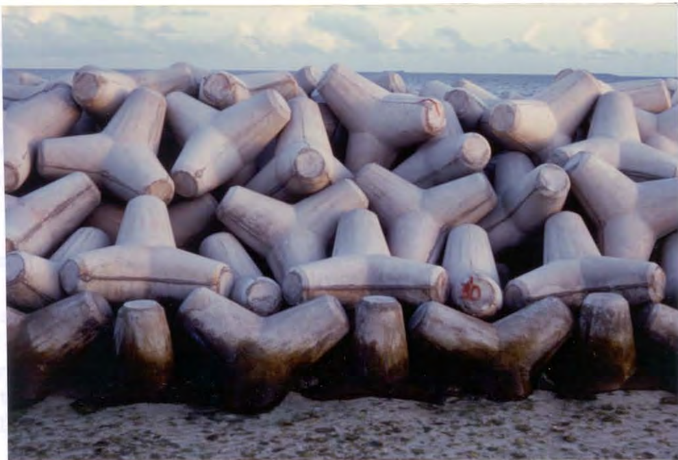
FIGURE 26. Face on view of one of the ten detached breakwaters on the south coast of Male' to show arrangement of the 3 tonne tetrapod armour units.
