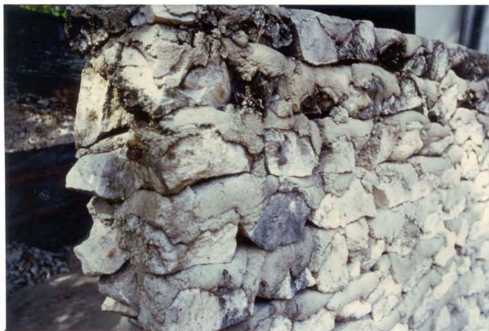
FIGURE 29. Close-up of a coral built wall. Note the large quantity of mortar required to bind the irregular coral nodules together.
