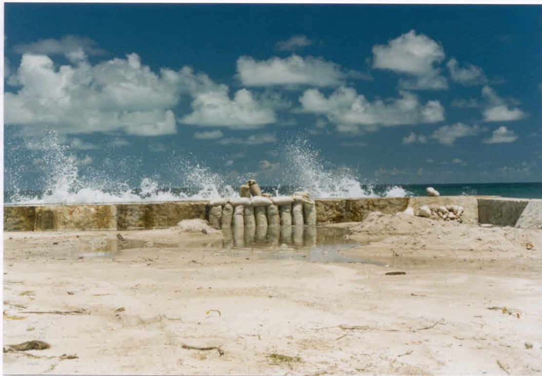
FIGURE 20. Retaining wall at south end of Hulule (marked A on Fig. 19) on a relatively calm day at high tide. Even in these conditions spray splashes over and water pools on the inside.
