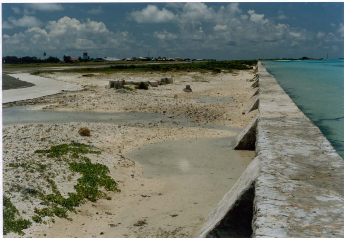
FIGURE 21. Retaining wall by south turning apron of Male' International Airport runway (marked B on Fig. 19). The toe of the wall is eroded so that seawater passes underneath at high tide, lapping right to the runway edge.
